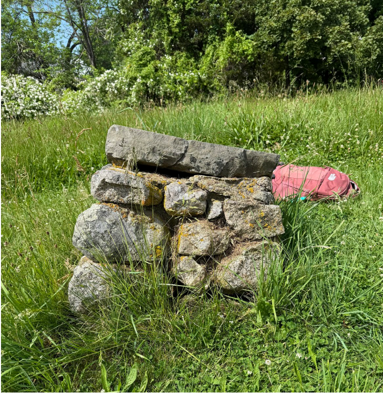
Figure 8 East-facing side edge of slab showing the rough-hewn dressing and the slope of the courses of fieldstones underneath it.
