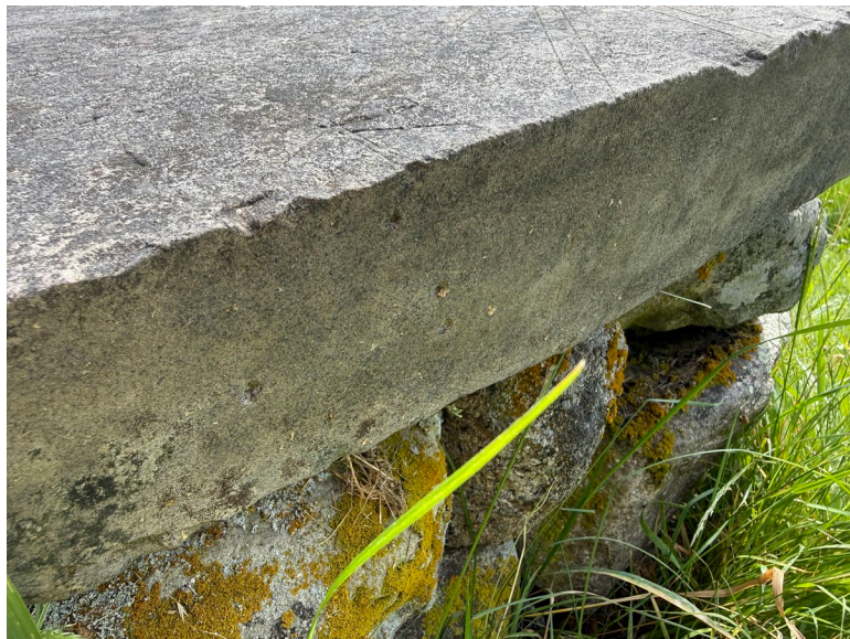
Figure 6 West-facing side edge showing flatness of finish.
