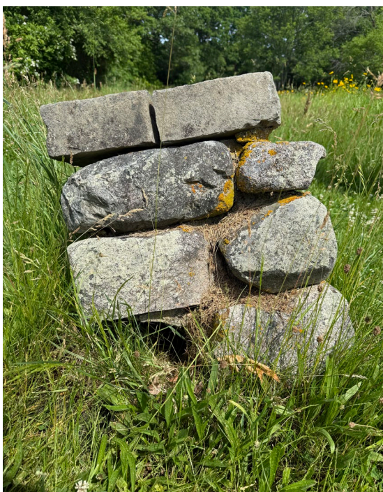
Figure 7 South-facing side edge of slab sitting atop fieldstone courses, showing the finish and slope.
