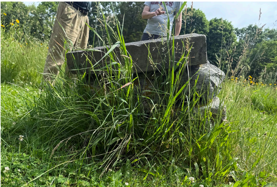
Figure 9 North-facing side edge showing the slope.
