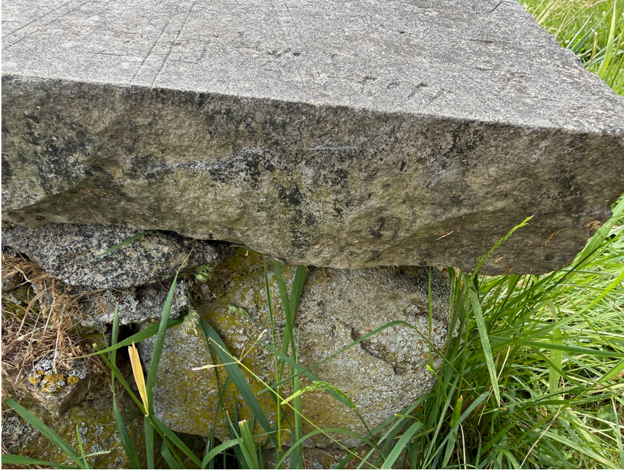
Figure 10 North-facing side edge detail.
